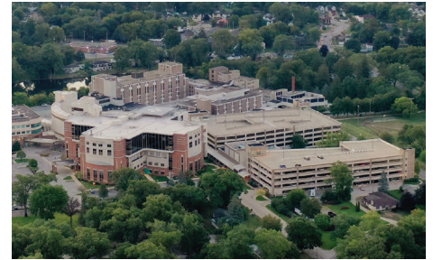
Elkhart General Hospital
