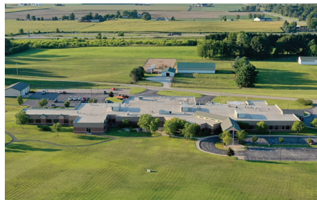
Community Hospital of Bremen
